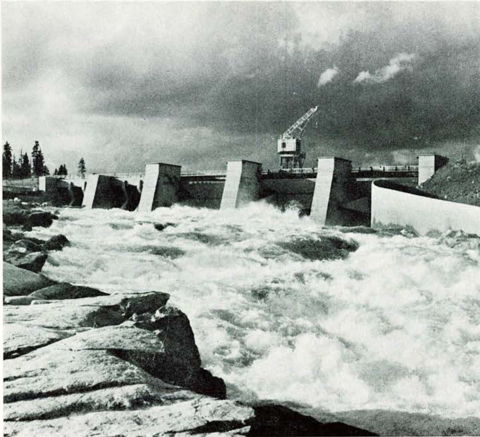
The economic hydroelectric potential of the Lule river basin in the north of Sweden is estimated at 14.6 million kWh per year. Above is one of the dams built to harness this energy.
