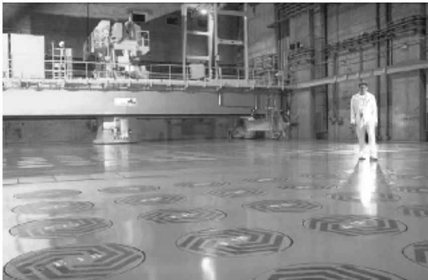
Figure 9.1. Vitrified waste interim storage room (Source: COGEMA – France)
