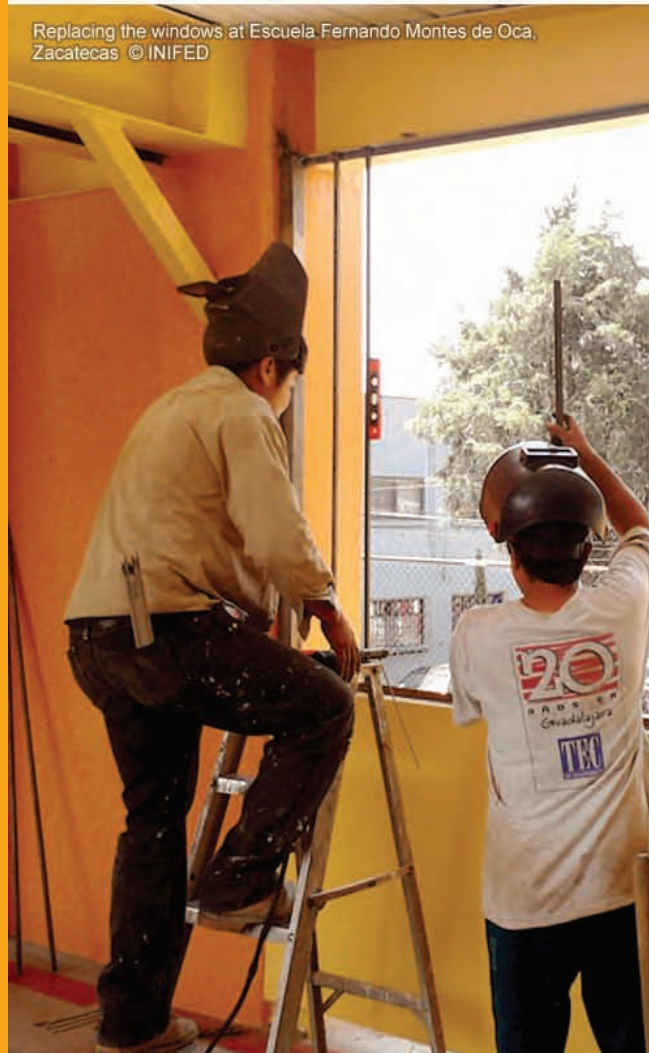
Carrying out work on a kindergarten roof © INIFED
