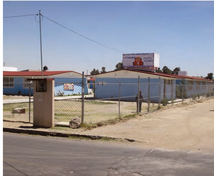
■ Figure 3.6 ■ Security fencing, Escuelas José María Morelos, Puebla © Alastair Blyth
