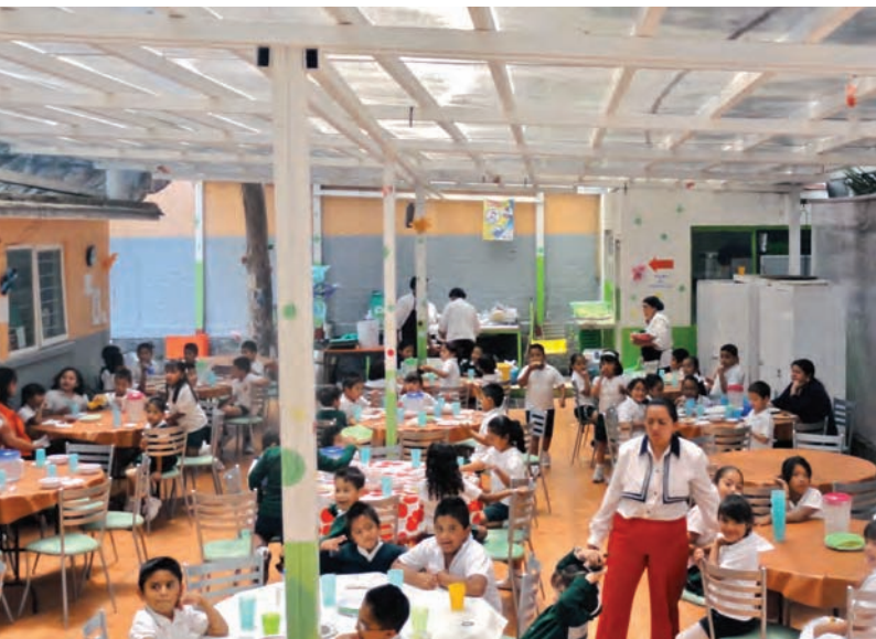
Figure 3.7 Polycarbonate roof at the Amistad Mundial School, Mexico DF
