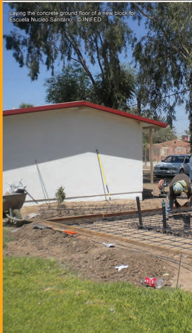
Laying the foundations for a better school - © INIFED
