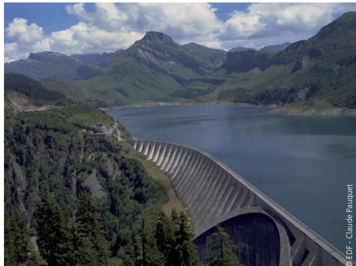
The EDF Roselend Dam in the Alps
