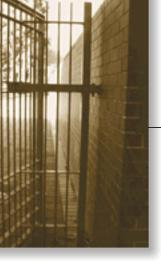
Fencing can be a "natural ladder" giving unwanted access to the roof
